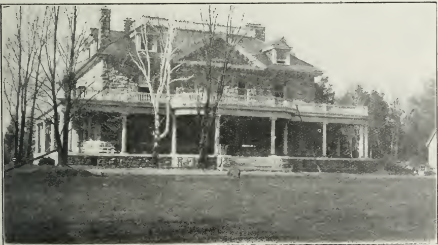
ROCKLIFFE PARK THE RESIDENCE OF WARREN V. SOPER, ESQ., OTTAWA
